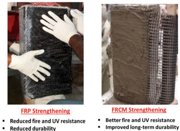
Fig. 3 Schematic representation of the advantages of FRCM over FRP
