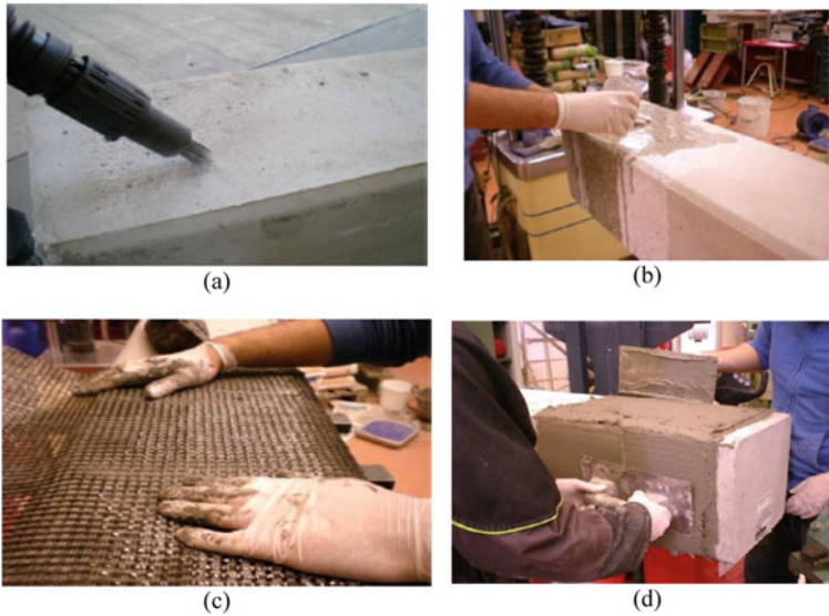
Fig. 7 Strengthening using FRCM system. a Surface preparation; b surface wetting; c FRCM application and d finishing (Picture Courtesy Escrig et al. 2015)
