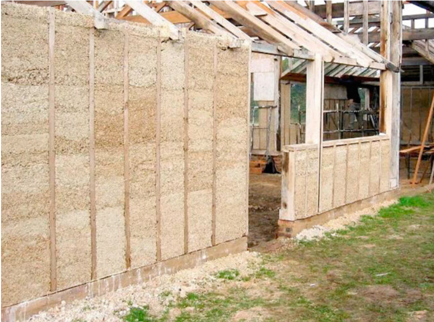
Fig. 7 Hemp line concrete walling(Steffens et al. 2017)
