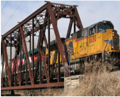
(a) Truss bridge
