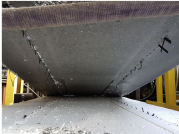
Fig. 33 The condition of the trussed grid connected when the top wythe is lifted after failure of the panel (O’Hegarty et al. 2019)
