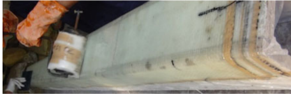
(b) Compaction the layers of fiber over mould
