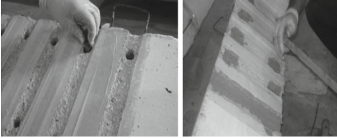
Fig. 5 Shear strengthening of beams using embedded connector system (Alam et al. 2017; Alam and Riyami 2018)
