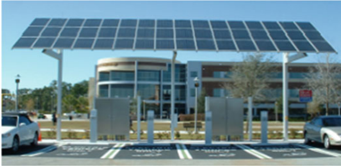
Fig. 1 PV-based parking lot for EV charging [6]
