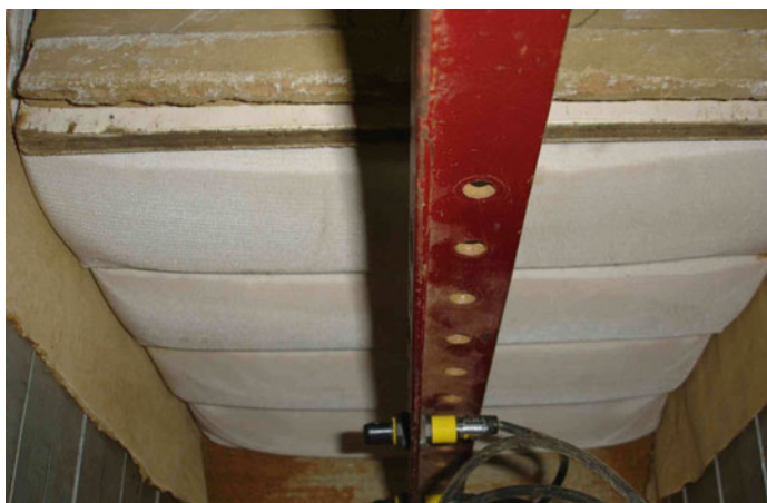
Fig. 15.1 Wrap-faced retaining wall built inside a laminar box. a Schematic diagram. b Photograph
