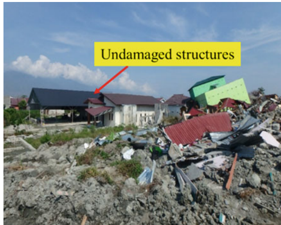
Fig. 12.31 Damaged and undamaged structures (Kiyota et al. 2020)
