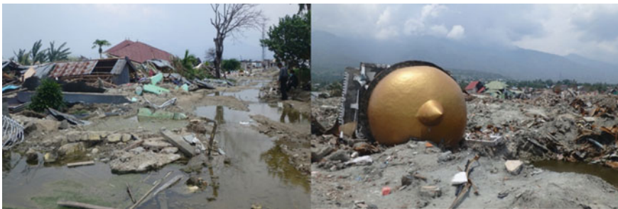
Fig. 12.26 Inundation of water after the earthquake and destroyed mosque structure due to the flow-slide (Kiyota et al. 2020)
