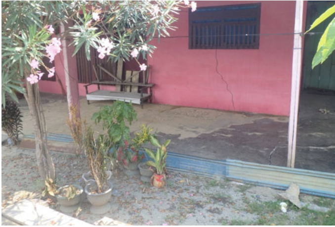
Fig. 12.27 Sand ejecta observed in the upper part of the flow-slide (Kiyota et al. 2020)
