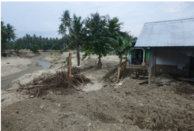
Fig. 12.11 Mud inundation mark on the house depicting the height of mud flow passing the area (Kiyota et al. 2020)
