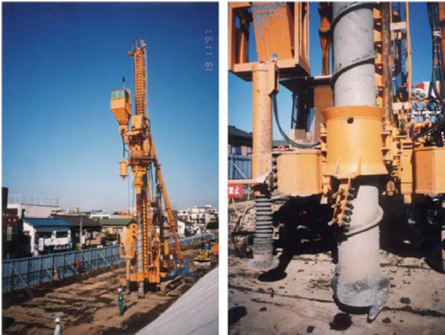
Fig. 3.17 Installation of gravel drains
