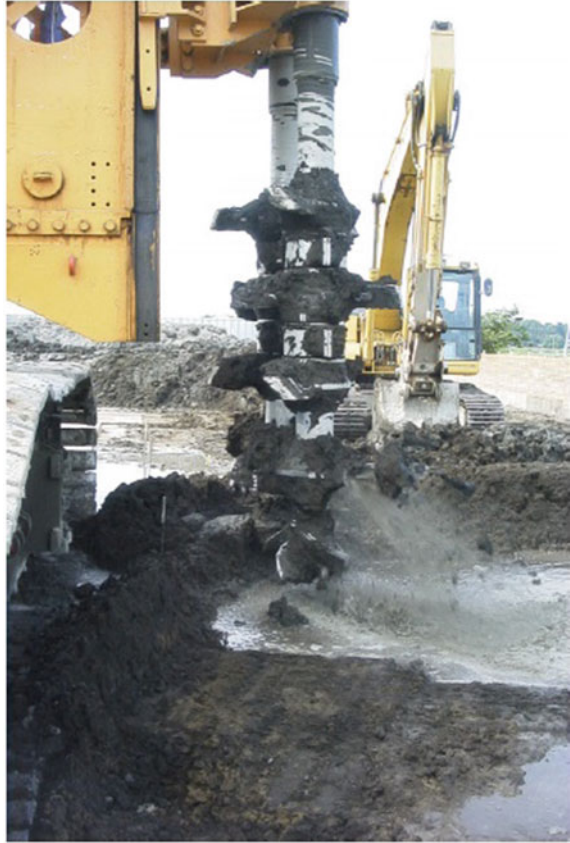
Fig. 3.12 Ongoing grouting by mechanical mixing
