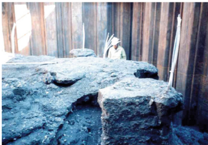
Fig. 3.28 Mass of sand solidified by injection of colloidal silica
