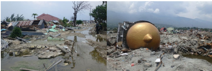
Fig. 12.26 Inundation of water after the earthquake and destroyed mosque structure due to the flow-slide (Kiyota et al. 2020)
