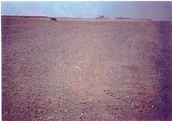
Fig. 3.10 Mitigative effect of dynamic consolidation in Lukang of Taiwan demonstrated during the 1999 Chi-chi earthquake (Kaiyo Kogyo Company)
