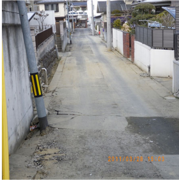
Fig. 3.44 Sand ejecta in residential embankment in hilly terrain near Sendai after the 2011 Tohoku earthquake (sand still remaining on road surface 17 days after the earthquake)
