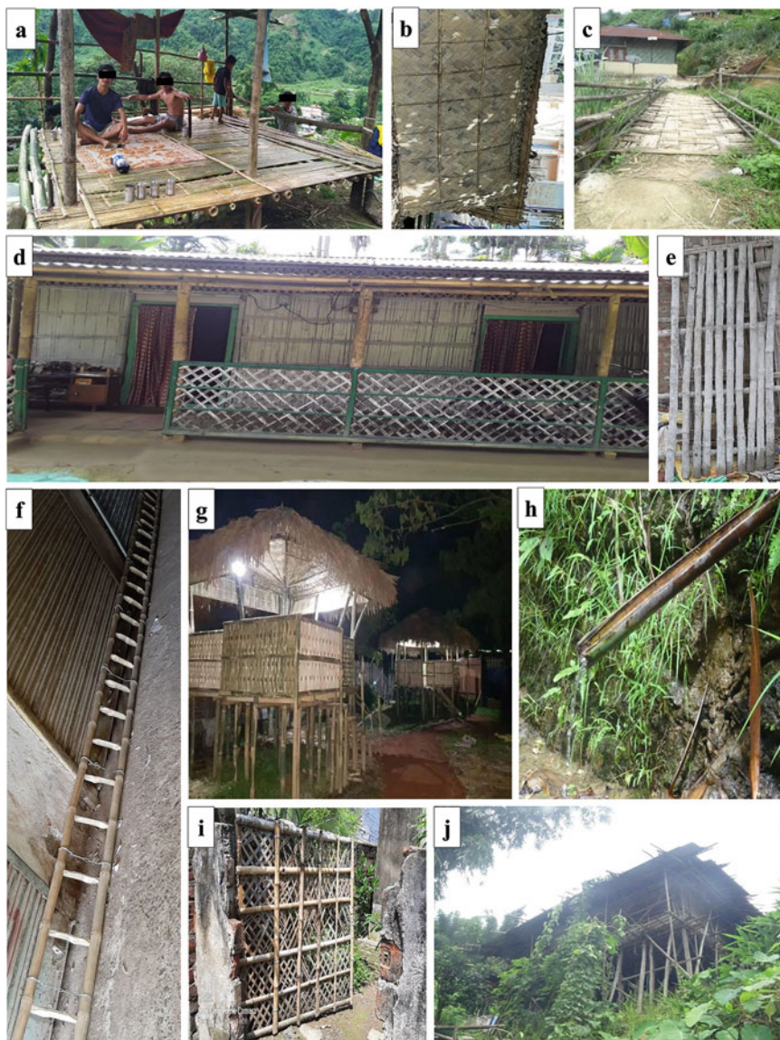
Fig. 14.5 Uses of bamboos for diverse constructional and allied purposes useful for ethnic lifestyle. (a) Community stage; (b) wall material ready to be fixed in a room; (c) bridge; (d) wall, fencing pillar of bamboo house; (e) bamboo float; (f) ladder; (g) bamboo-made house; (h) bamboo channel used for transporting water; (i) bamboo gate; (j) bamboo poles used as supporting pillars of a hanging house. (a, b, c, e, f, g, h, i, and j) were obtained from the Nyishi tribal community of Senki view, Itanagar, Arunachal Pradesh, and (b) from Boro tribal community of Kamrup, Assam, India
