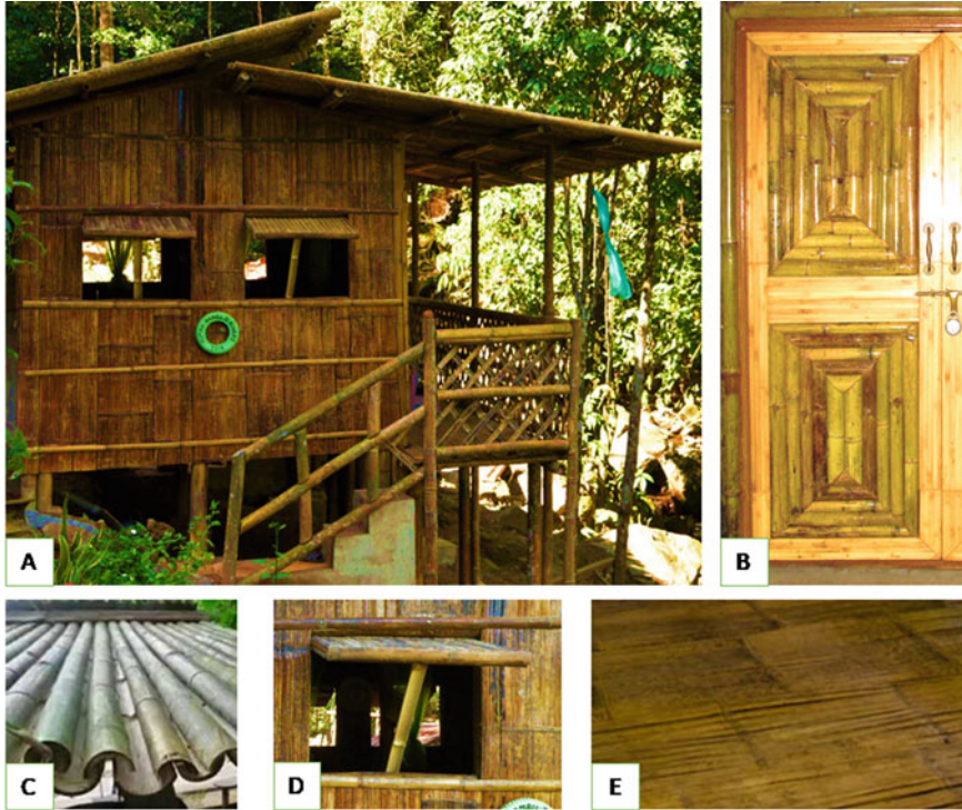
Fig. 20.3 Example of bamboo application in building construction. (a) Hut made entirely out of bamboo. (b) Bamboo door with wood frame. (c) Bamboo roof. (d) Bamboo window. (e) Bamboo floor
