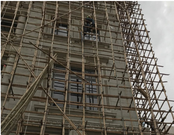
Fig. 20.5 Bamboo scaffolding
