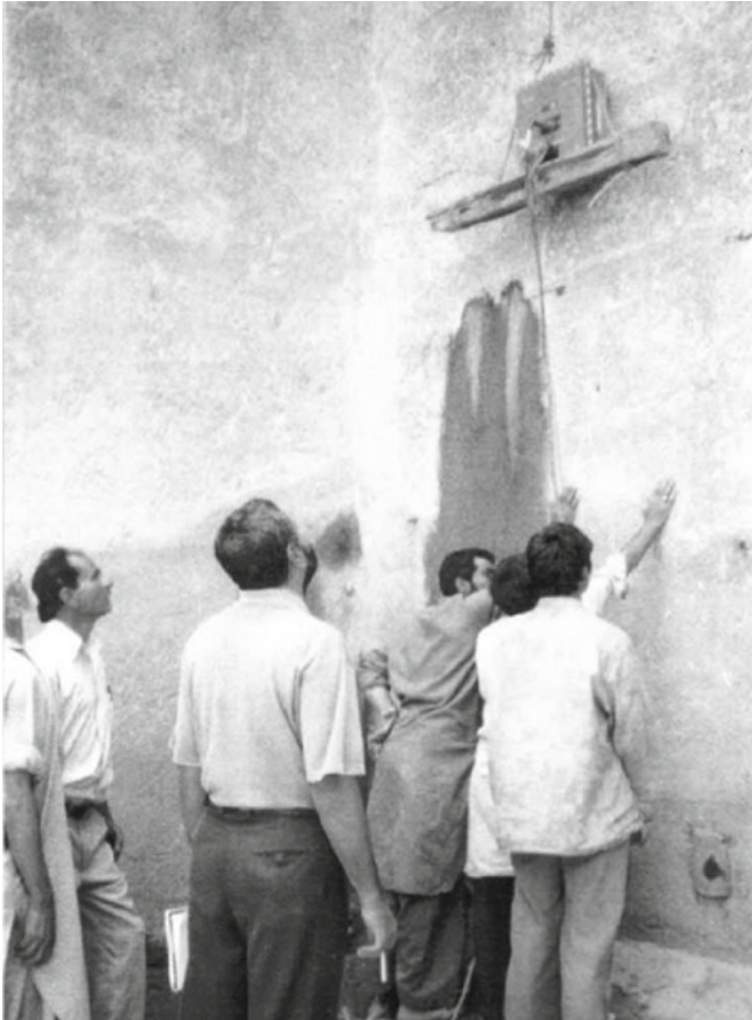
Fig. 6 Photograph of GPR scan on upstream face of Lower Jhelum Dam
