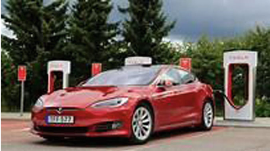
Fig. 11 Electric vehicle charging station
