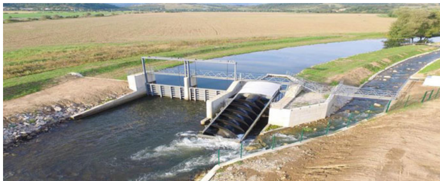
Fig. 3 Screw hydro turbine water dam
