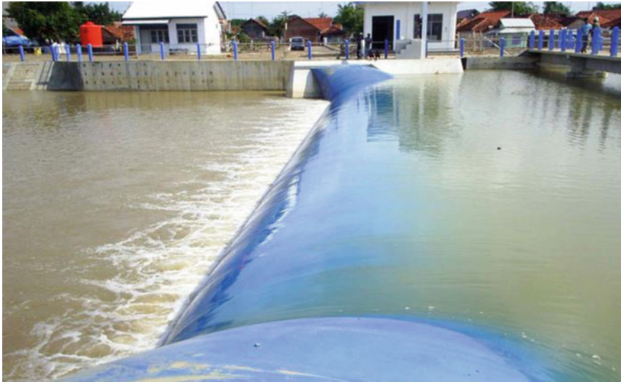
Fig. 6 Inflated rubber water dam
