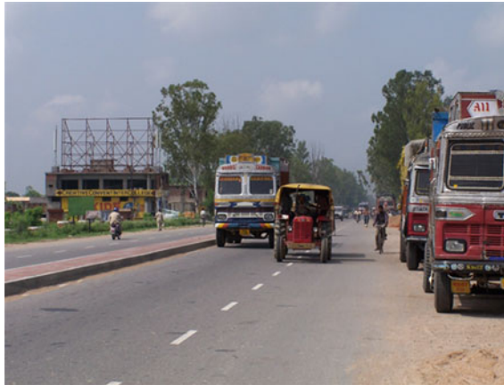
Fig. 6.3 Mixed traffic on a four-lane divided highway in India
