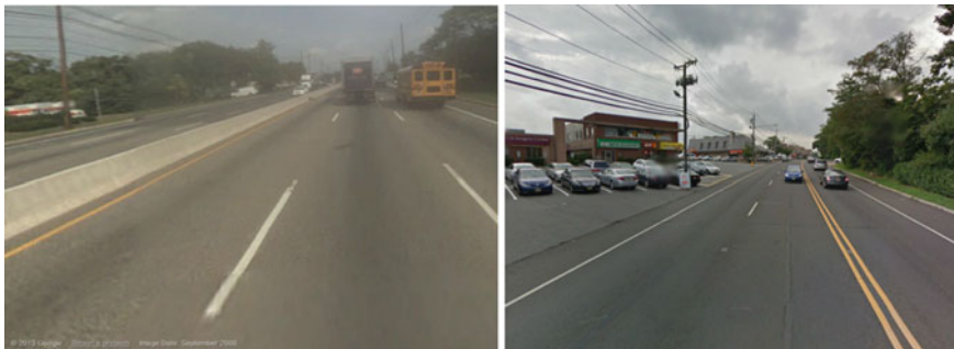
Fig. 9.7 High-speed arterials with no pedestrian infrastructure, (left image) US 130, Cinnaminson, Burlington County, NJ, and (right image) Bergen Boulevard (NJ 63), in Palisades Park Borough, Bergen County ( source Google Street View)
