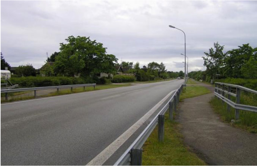
Fig. 7.3 Separation of pedestrians and cyclists on a street with high speeds and low use of the separation
