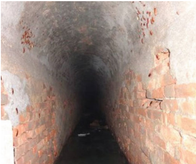
Fig. 2 Sewer tunnel in Saigon (in French colonies period) [7]
