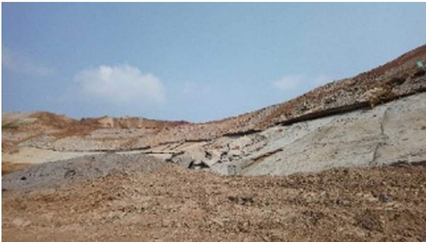
Fig. 2 A panoramic view of the landslide of Nhan Co
