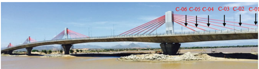
Fig. 4 An-Dong Bridge in Vietnam (source: picture taken by the 3rd author)
