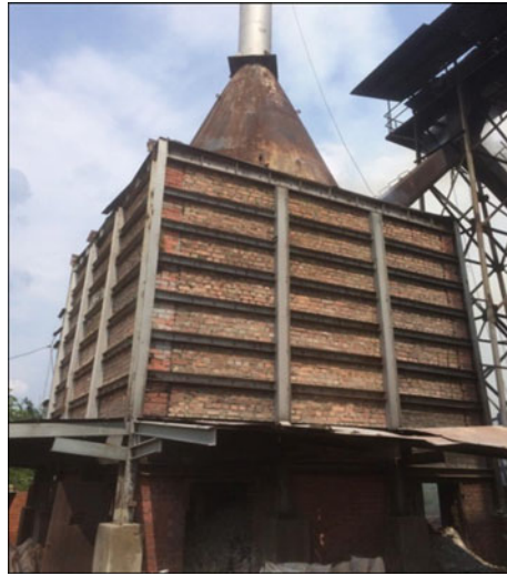
Fig. 2 Incinerator of the palm oil husk of fiber burning
