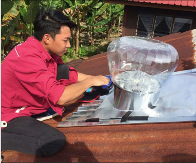
Fig. 4 Installation of PhotoVenti on an inclined roof
