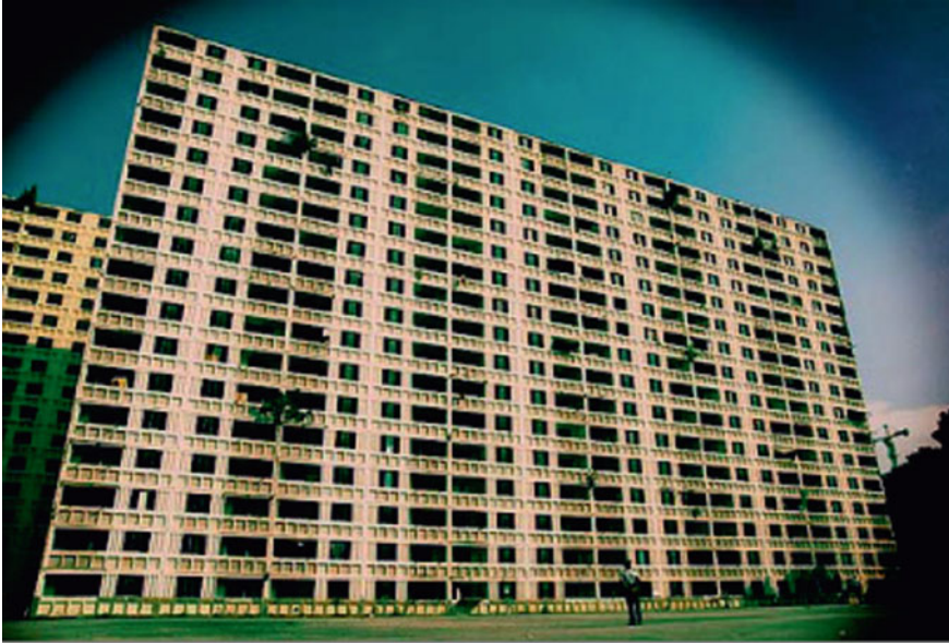
Fig. 1 IBS implementation in Pekeliling Flats, Kuala Lumpur [49]
