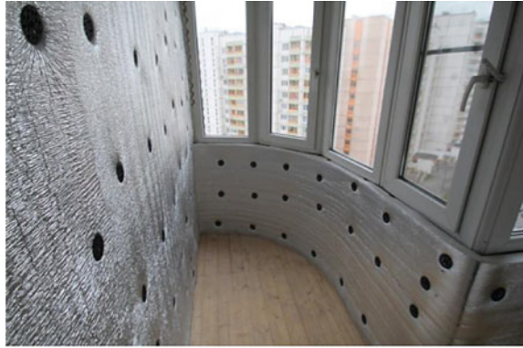
Fig. 22 Insulated loggia before the facing (owned by our company)
