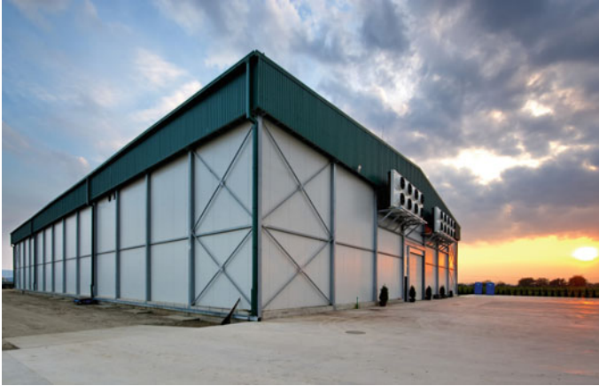
Fig. 5 Commercial refrigerator built on the base of single-floor storage (open sources, https://www.shutterstock.com/g/Aleksandar%20Milutinovic )
