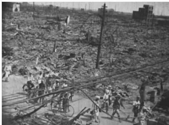
Fig. 13.1 Devastating damage by the Great Kanto Earthquake in 1923 (From "Actual damage by the Great Kanto Earthquake in Tokyo" Tambasayama City Audio-Visual Library)
