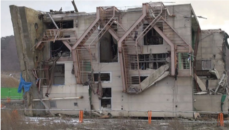
Fig. 5.2 Steel frame building (demolished)
