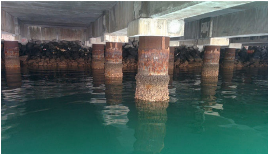
Fig. 3 Photograph of the arrangement of piles in the jetty
