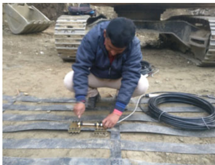
Fig. 7 Fixing the strain gauges with plates on primary reinforcement (geogrid) at the site for valley side reinforced soil system
