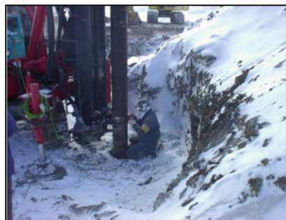
(d). Joint cutting.
