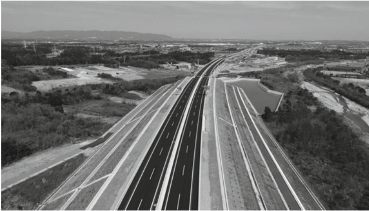
Photo 7 Embankment section of New Meishin expressway
