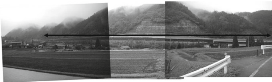
Photo 5 Embankment and cut sections of the pre-opened Tokai-Hokuriku expressway
