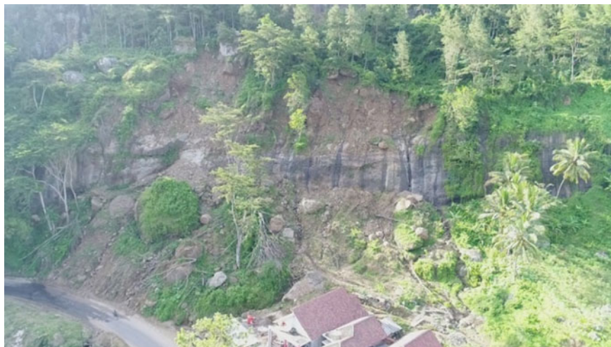
Fig. 2 Typical landslides along road cut slopes in Trenggalek
