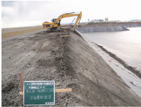
Fig. 7 Construction status of the extra fill on revetments near No.9
