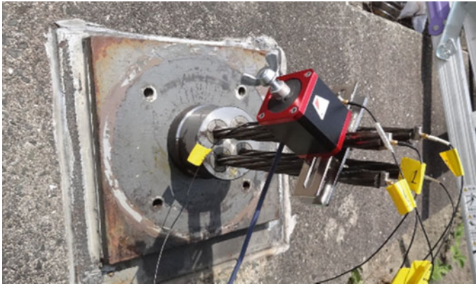
Photo 1 Small size vibrator attached on the extra length of anchor head
