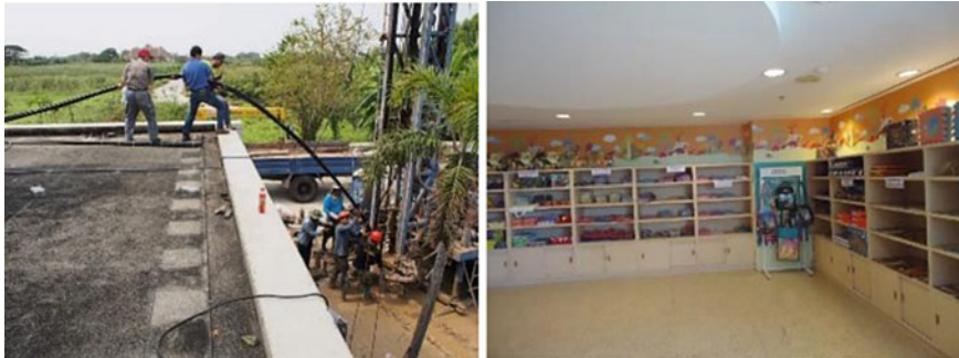
Fig. 8 Installation of GHE into the borehole (middle); museum's souvenir shop (right)
