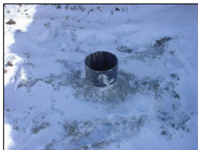
(a). Revealed pile head.
