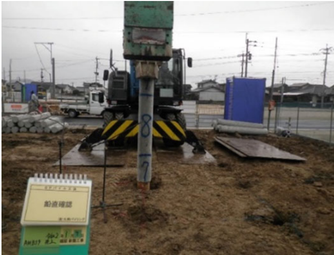
Fig. 2 Jointed-timber pile installation
