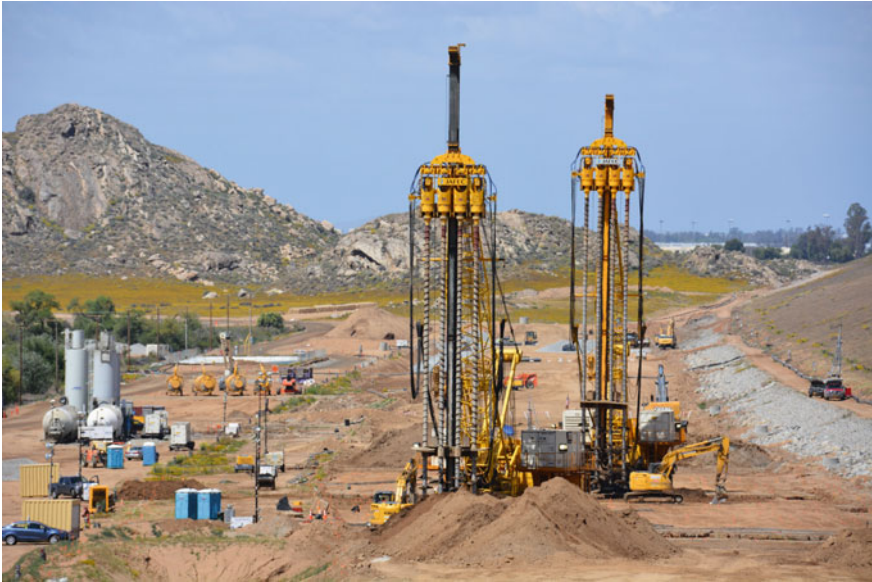
Fig. 3 DMM mixing equipment at Perris Dam Site
