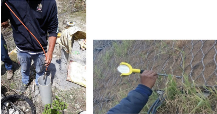
Fig. 8 Installation of inclinometer in the borehole (left-aligned) and reflectometer (right-aligned)
