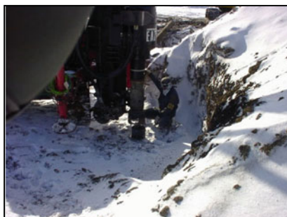
(b). Set pile head cap.
