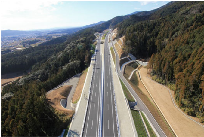
Photo 6 Embankment and cut sections of New Tomei expressway
