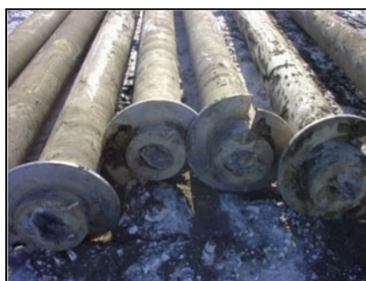
(f). Retrieved piles.
