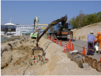
(a) Retrieved piles
