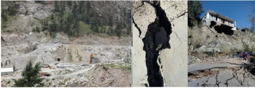
Fig. 10 Small range seismic waves due to blasting and tunnelling operations
