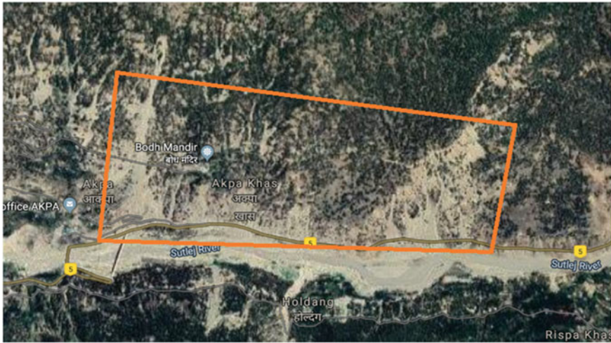
Fig. 2 Ribba village landslide zone [9]
