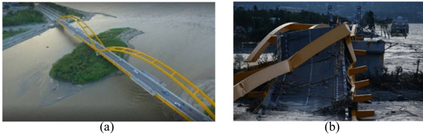
Fig. 6 Palu bridge IV a before the earthquake b after the earthquake [1]
