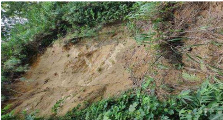
Fig. 8 Landslide area with less vegetation cover
