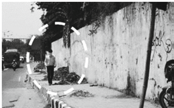
Fig. 4 Inadequate width of sidewalks
