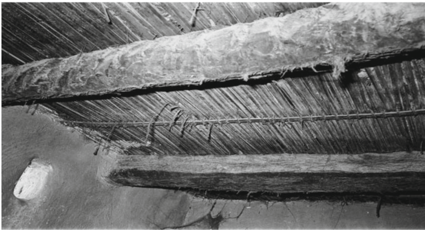
Fig. 92 Using date palm trunks as beams with date palm midribs ceiling in a simple roof, Arish, Egypt
