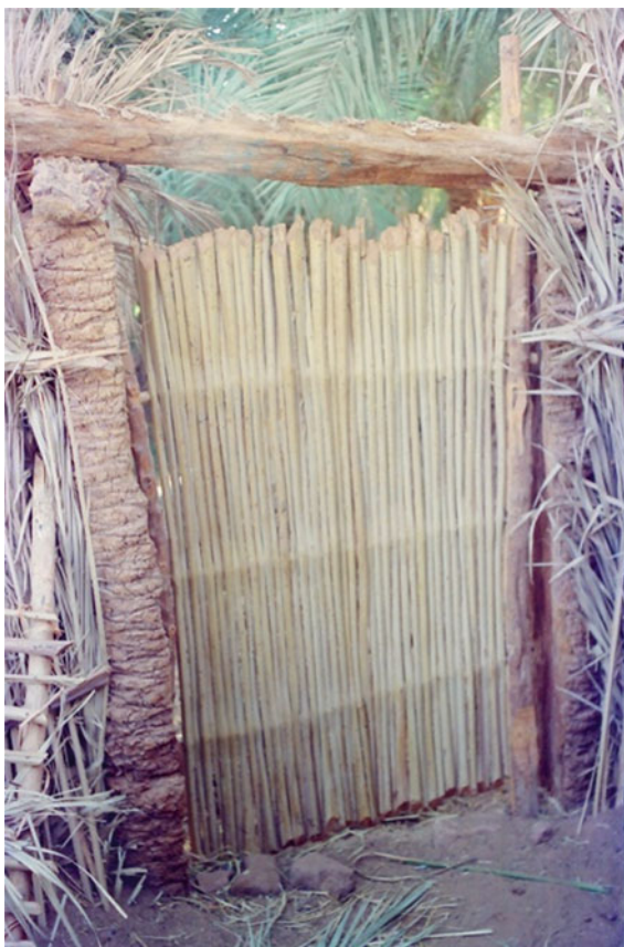
Fig. 41 A simple fence door made from pierced date palm midribs, New Valley, Egypt
