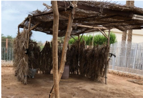
Fig. 22 Sheathing by whole date palm leaves over spadix stem nets supported by wooden poles
