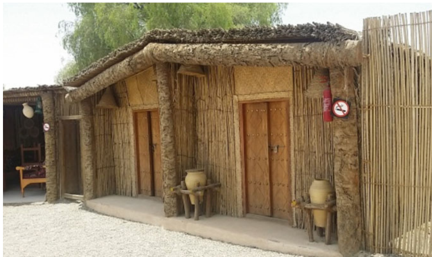
Fig. 94 Using date palm trunks as columns and rafters in a date palm midrib hut
