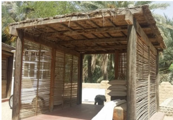
Fig. 96 Squared date palm trunk beams and columns in a modern date palm midribs hut
