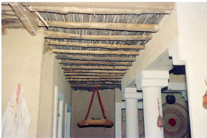
Fig. 30 Roofing using palm midribs over a series of tree branches as beams, Fayoum, Egypt
