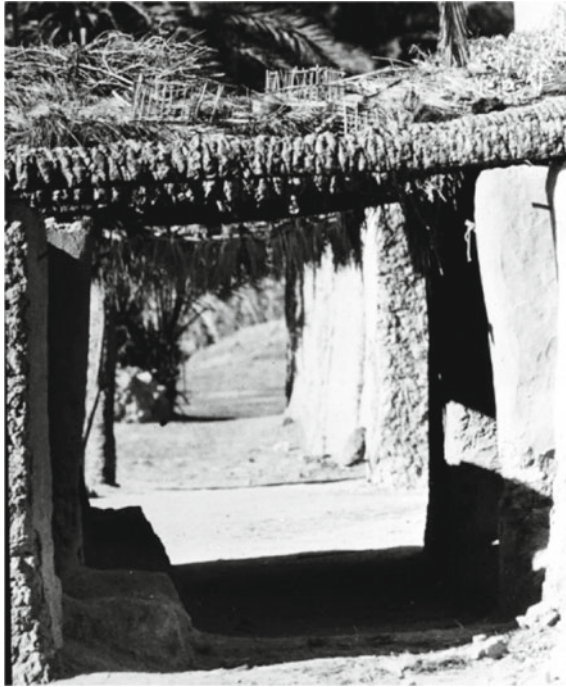
Fig. 91 Using date palm trunks as beams in an outdoor corridor, Arish, Egypt
