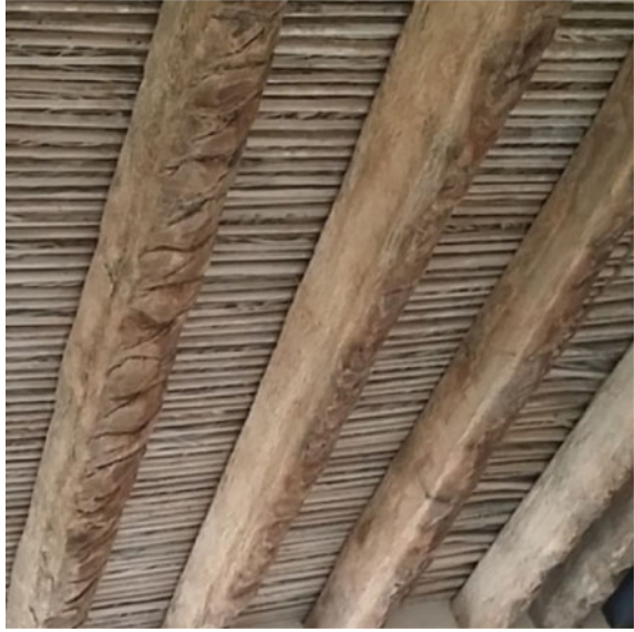
Fig. 95 Quartered date palm trunk beams that support date palm midribs roof
