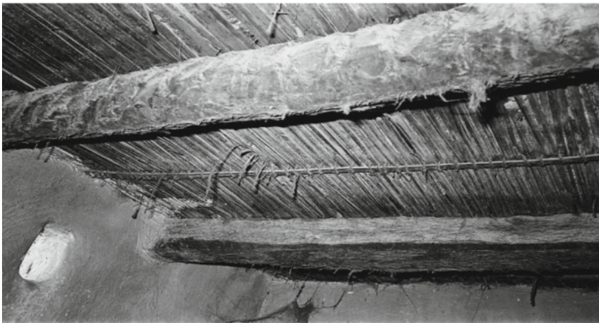
Fig. 92 Using date palm trunks as beams with date palm midribs ceiling in a simple roof, Arish, Egypt
