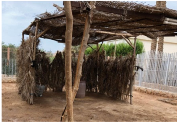
Fig. 22 Sheathing by whole date palm leaves over spadix stem nets supported by wooden poles
