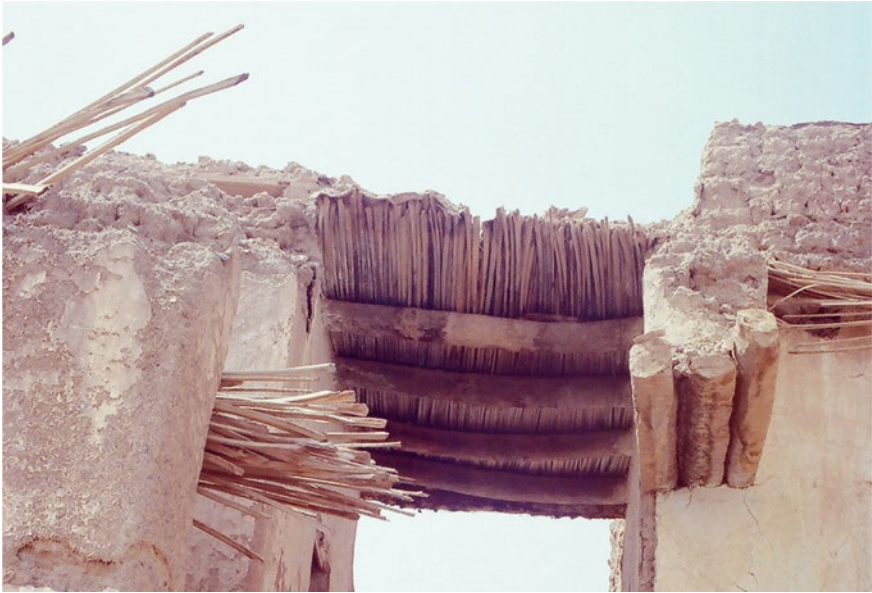
Fig. 31 Ceiling of an outdoor corridor made of date palm midribs supported by wooden planks, North Sinai, Egypt
