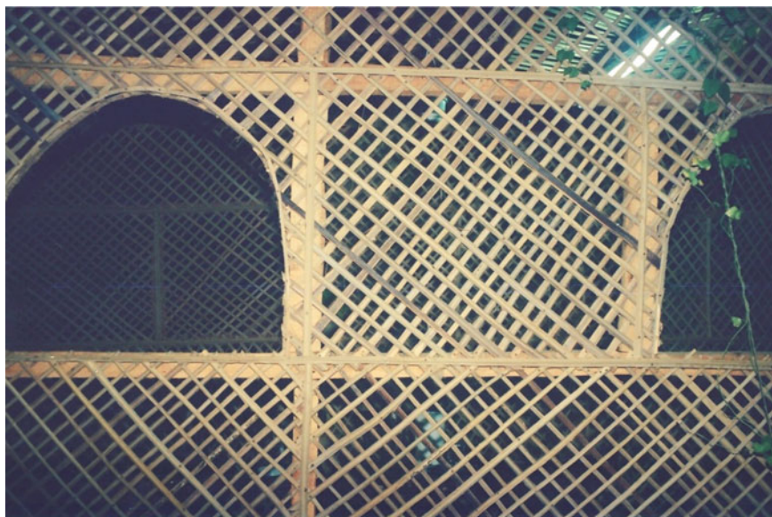
Fig. 36 Diagonal date palm midribs lattice in an outdoor fence, New Valley, Egypt
