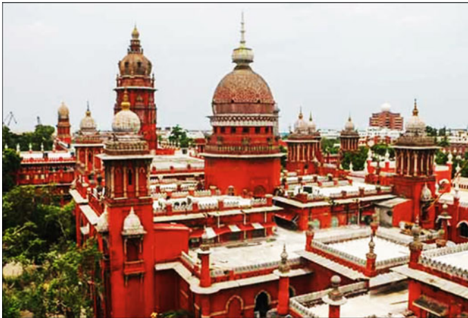
Fig. 1 Madras high court building, Chennai, Tamil Nadu [9]
