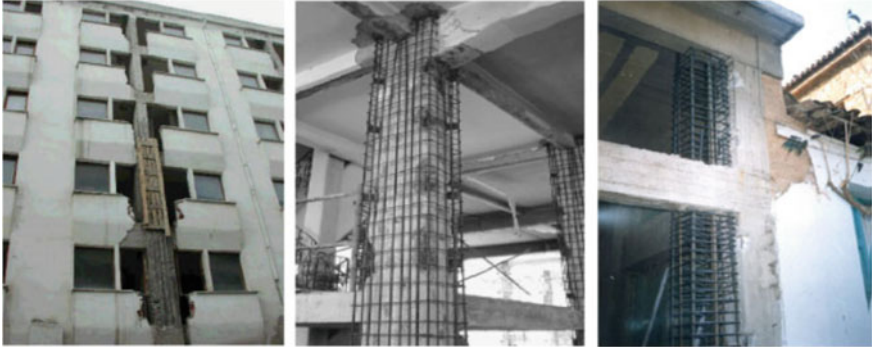
Fig. 5 Reinforced concrete (RC) jacketing applied through several floors [22]
