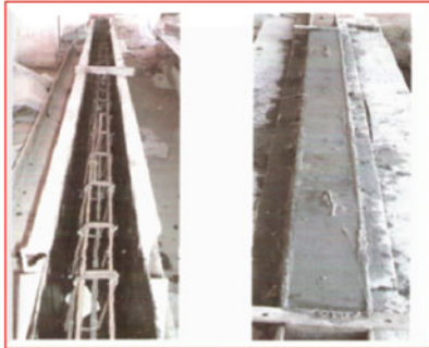
Task 1: Casting of concrete beam specimen
