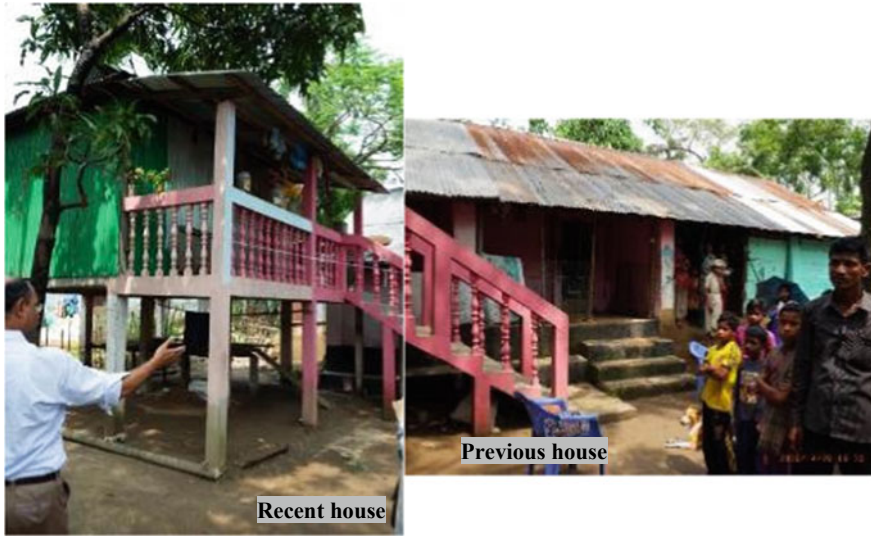
Fig. 14.14 A house with the floor raised higher (left) and the original structure with traditional plinth (right), Goainghat, Sylhet, April 2017
