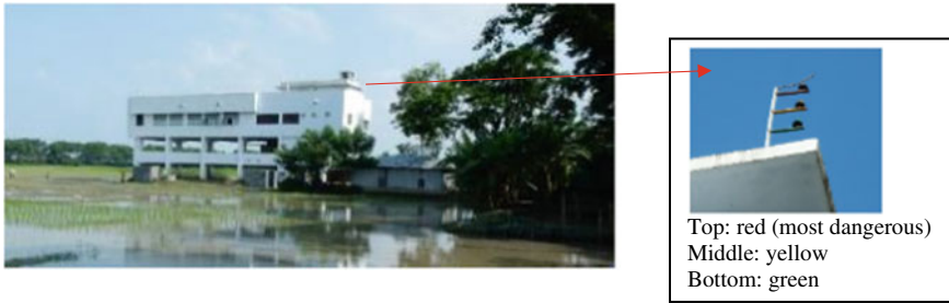
Fig. 14.15 A cyclone shelter houses both livestock (first floor) and people (second floor). A warning system with lights that signify levels of danger has been installed. Sarankhola, Bagerhat District, Khulna Division, August 2014
