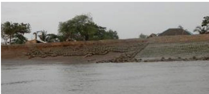
Fig. 14.12 Sand bags and concrete blocks are placed on the embankment to prevent erosion (Fulchhari District, Gaibandha Division, 2014)
