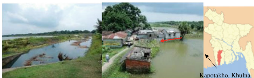
Fig. 14.6 Poor polder drainage (left) and sedimentation resulted in inundations marked by levels of discoloration in buildings (middle) (Kapotakho in Khulna District, 2014)
