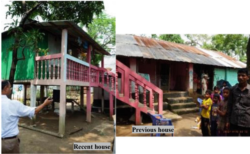
Fig. 14.14 A house with the floor raised higher (left) and the original structure with traditional plinth (right), Goainghat, Sylhet, April 2017
