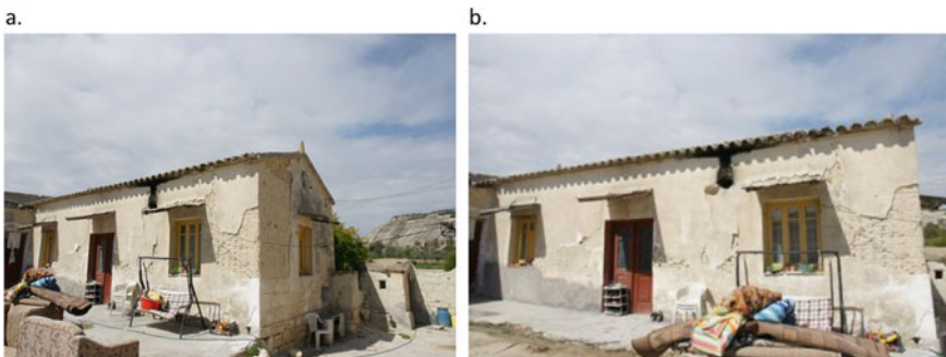
Fig. 6 Case study building [16]
