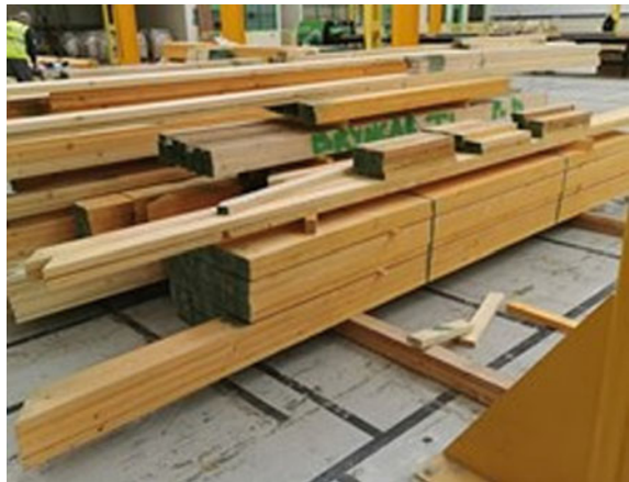
Fig. 13 Stacks of cut timbers arranged into truss types ready for assembly. The smaller timbers (webs) can be seen on the top of the stack, whereas the larger timbers (TCs and BCs) which are accessed first can be seen on the bottom of the stack (authors image 2019)
