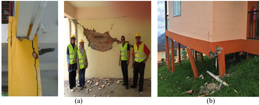
Fig. 12.2 Damage to buildings due to Ranau Earthquake a shear failure at residential, b column failure at rest house
