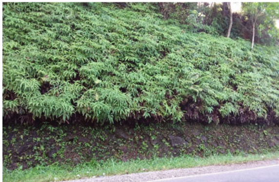
Fig. 16.14 Native mono-culture vegetation on overburdened soil standing above the completely weathered rock in Avissawella — Nawalapitiya road
