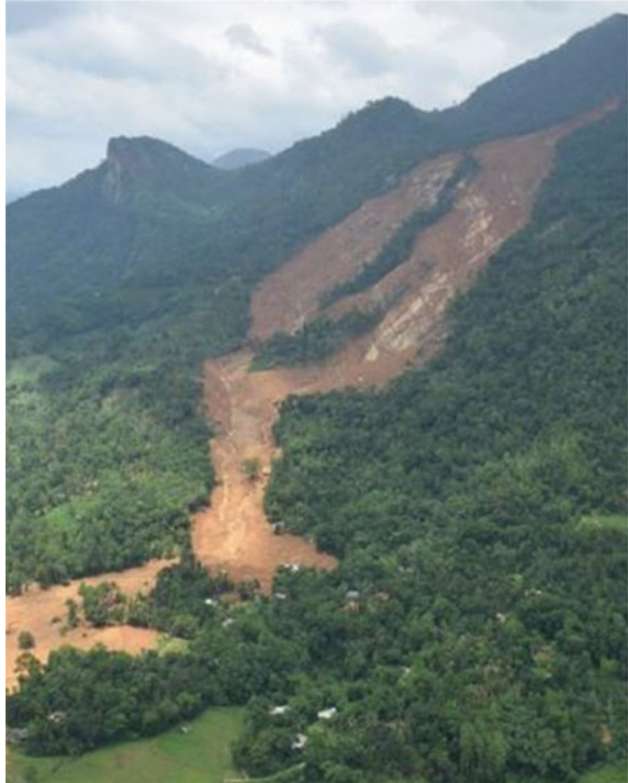
Fig. 16.7 Landslide event captured more than 127 victims in Aranayake, Kegolle district in Sri Lanka (JICA 2016)
