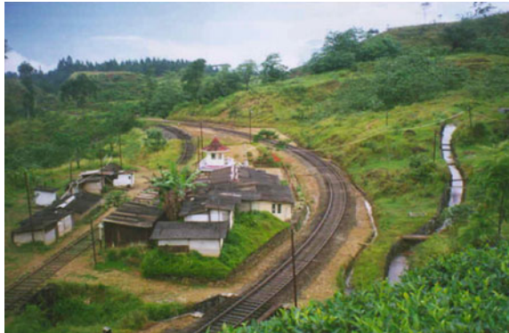
Fig. 15.15 Present situation at Watawala after mitigation
