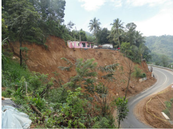
Fig. 15.8 A non-engineered housing construction
