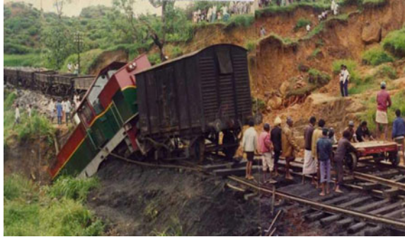
Fig. 15.14 Damage to the railway track
