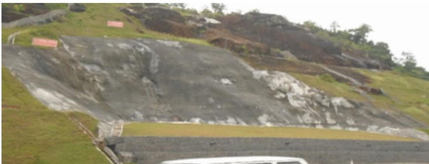
Fig. 15.27 Slope at southern expressway after mitigation
