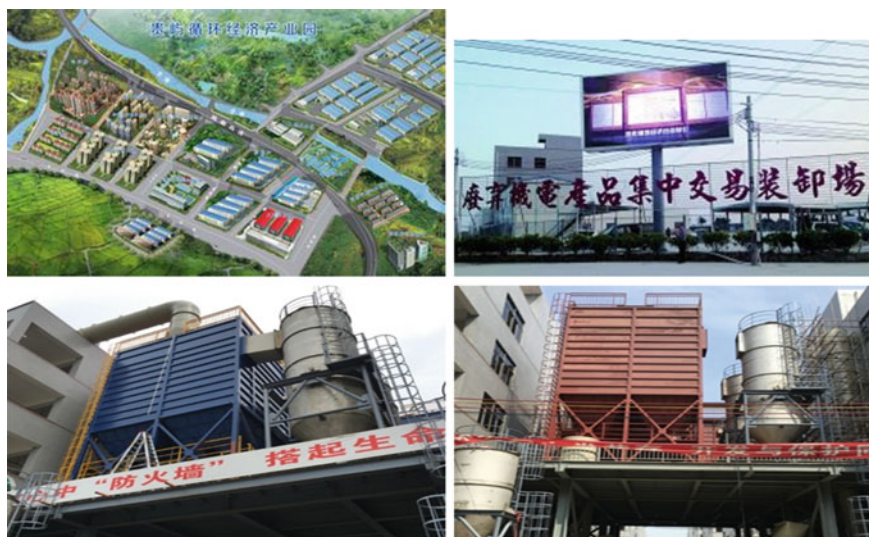
Fig. 13 Park flue gas treatment equipment (The first picture is from the following website https://www.sohu.com/a/164860752_99908715 . The second picture is from the following website. http://sn.people.com.cn/big5/n2/2016/0113/c340887-27533674.html )
