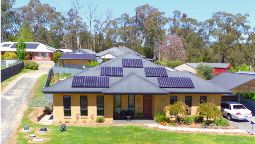
Fig. 9 Yackandandah community microgrid in Victoria, Australia
