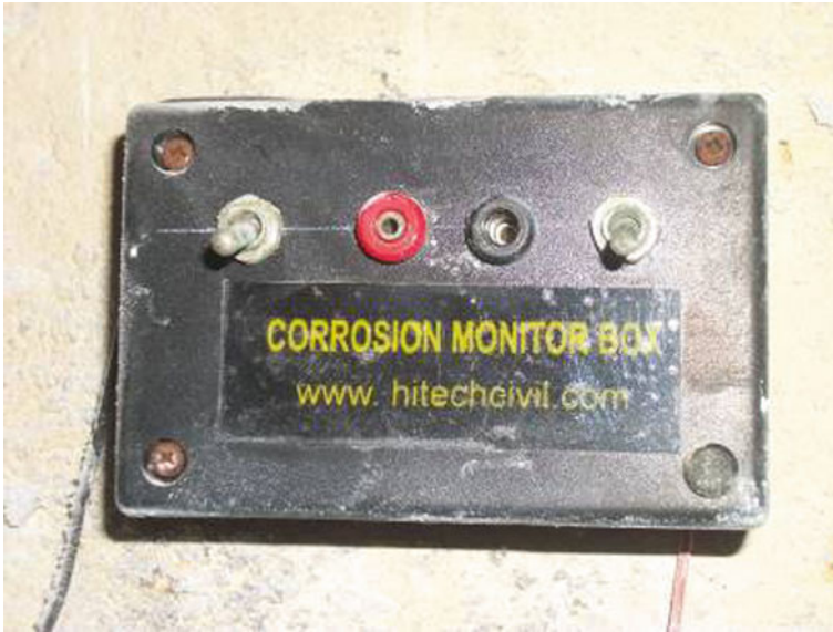
Fig. 14 View of the corrosion monitoring box
