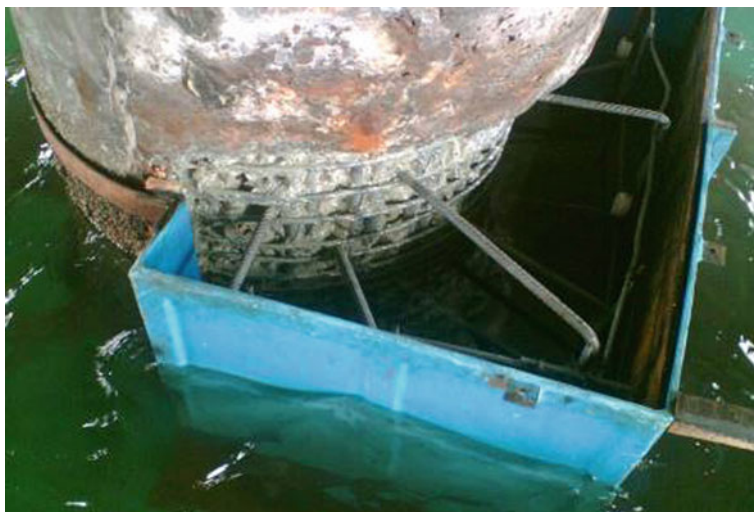
Fig. 13 View of positioning of Galvanic anode, form work and jointing compound
