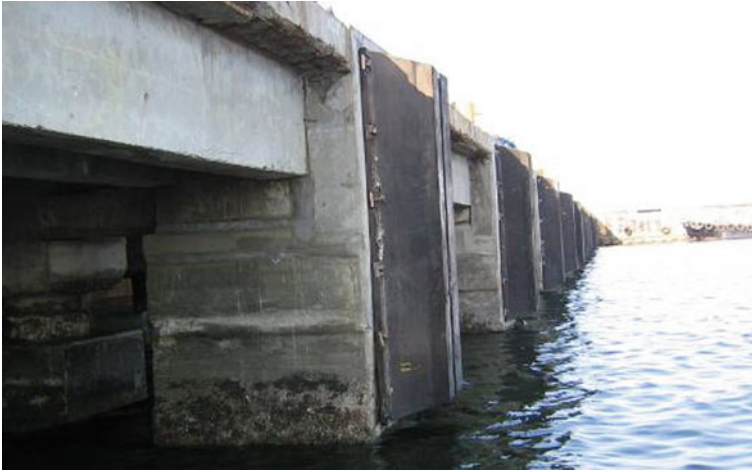
Fig. 15 Complete view of the jetties after jacketing with under water micro-concrete
