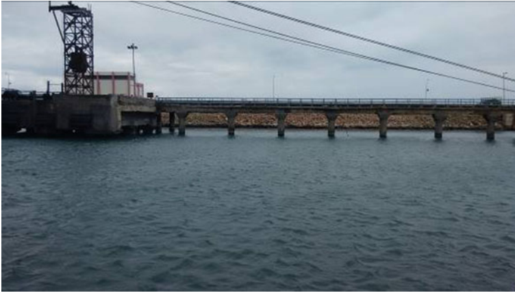
Fig. 7 View of the coal jetties at VOC Port
