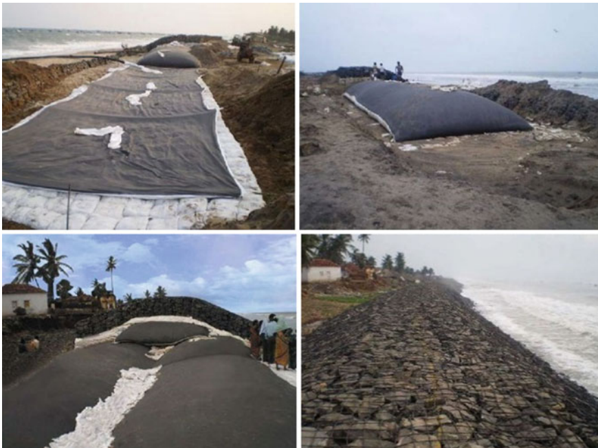
Fig. 6 Construction stages of seawall at Uppada, Andhra Pradesh [24]
