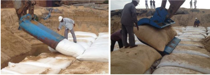
Fig. 7 Coastal protections using geobags in Ullal, Karnataka [4]
