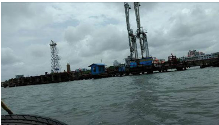
Fig. 3 A view of the STB jetties of M/s BPCL at M/s Cochin Port Trust, Kochi
