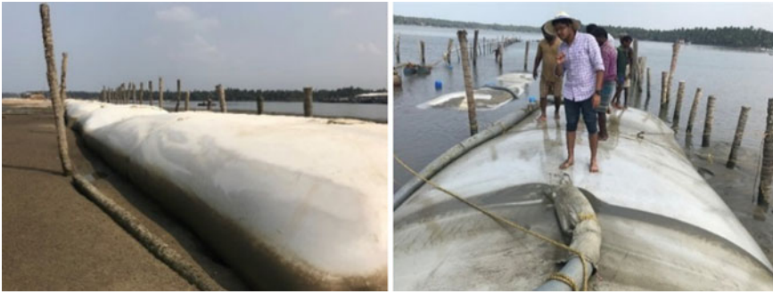
Fig. 9 Geotube Island reclamation, Cheruvattor, Kerala (photographs taken during field visit)
