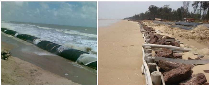
Fig. 1 Geotextile tubes at Shankarpur [21]
