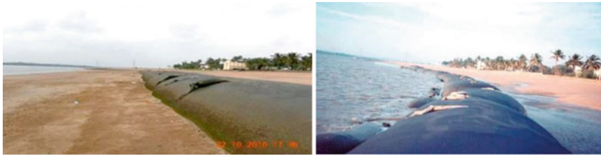
Fig. 3 Geotextile reef at INS Hamla, Maharashtra [22]
