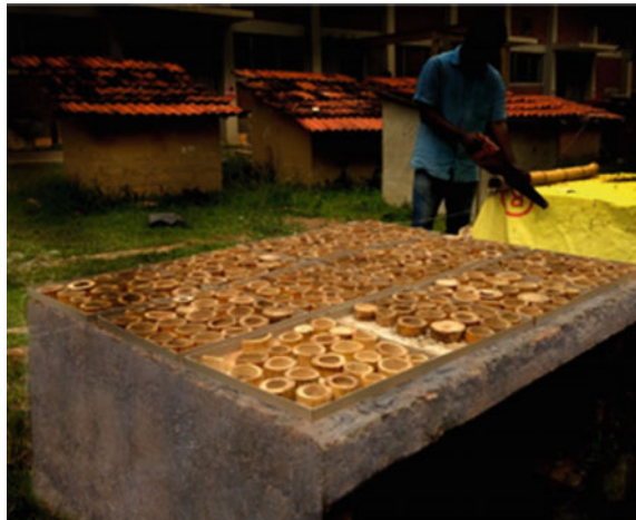
Fig. 17 Bamboo insulated concrete slab system [52]
