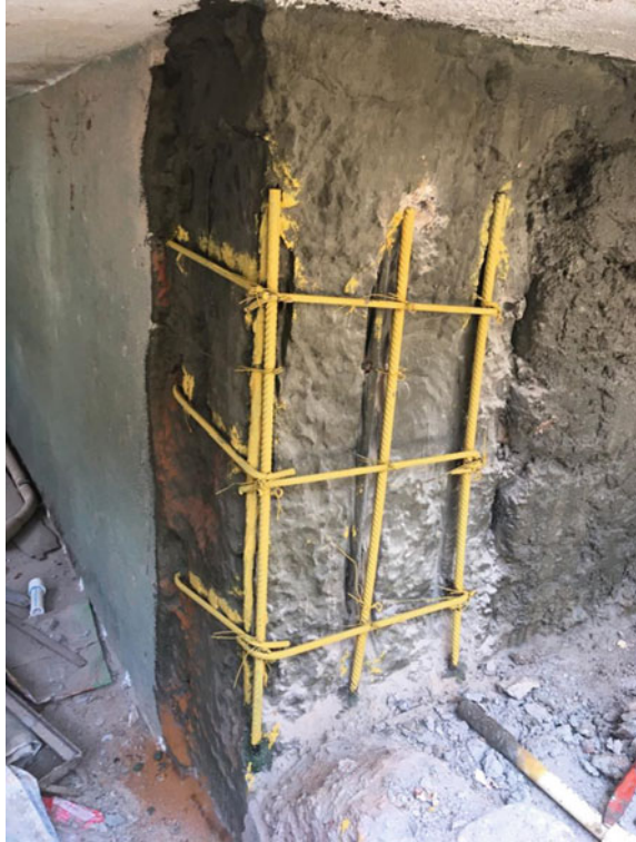
Fig. 7 Coating of Steel bars
