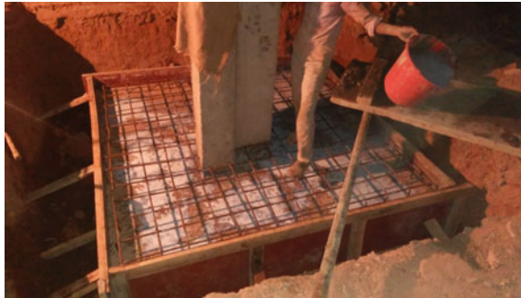
Fig. 2 Steel Reinforcement at footing top
