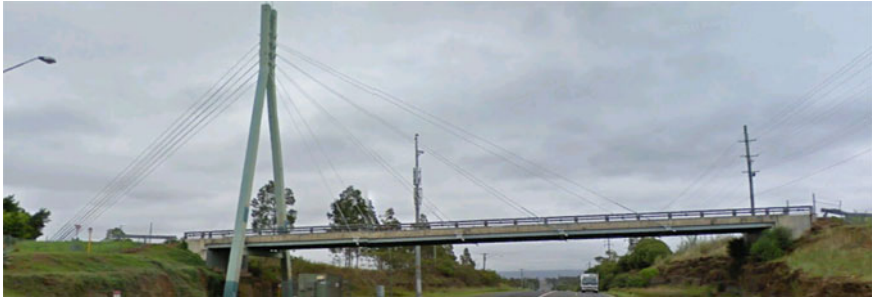
Fig. 5 Cable-stayed bridge for tests
