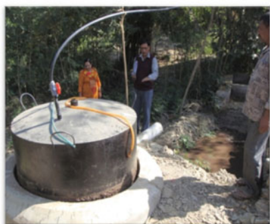
Fig. 4 Modified KVIC biogas plant for Aloe vera waste installed at beneficiary site
