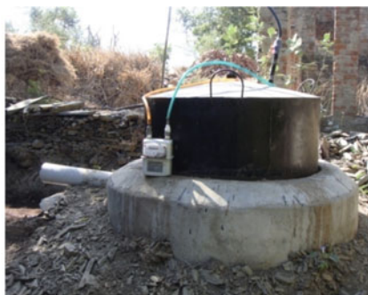
Fig. 4 Modified KVIC biogas plant for Aloe vera waste installed at beneficiary site
