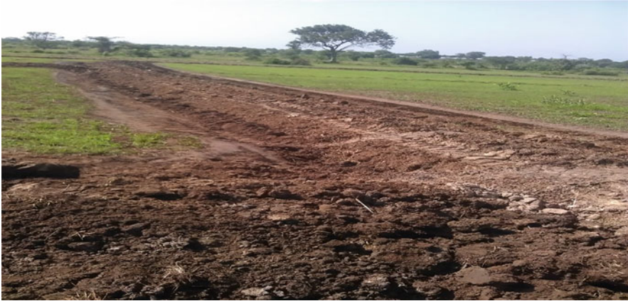
Fig. 11.7 Bund created for water control measure
