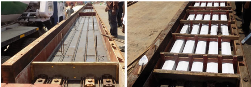
Fig. 3 Various stages of prestressed HCS specimen casting
