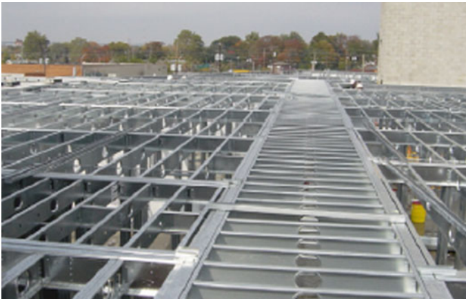
Fig. 1 Lipped channel beams as floor joists [18]
