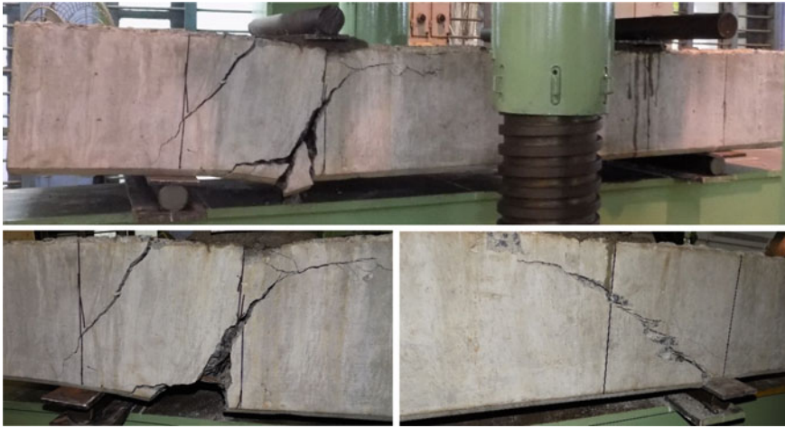
Fig. 11 Tested specimens with shear cracks
