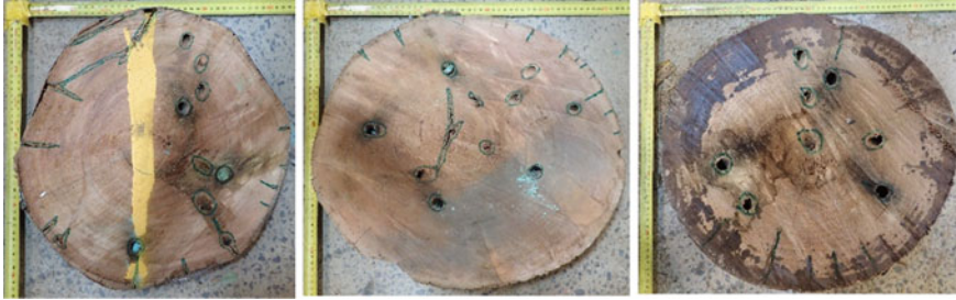
Fig. 5 Reduction in cross-sectional area due to multiple drill holes in sectioned timber pole specimens
