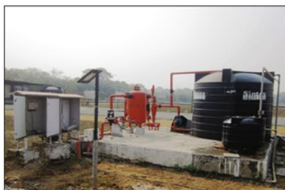
Fig. 15.17 Control head and setup of drip irrigation system
