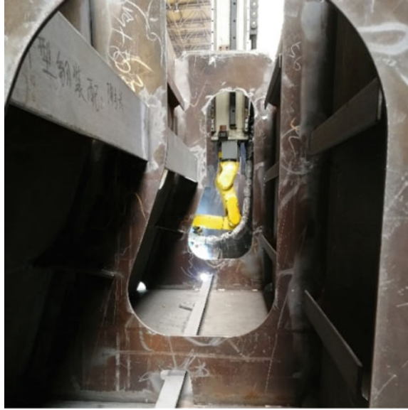
(a) Robot vertical welding
