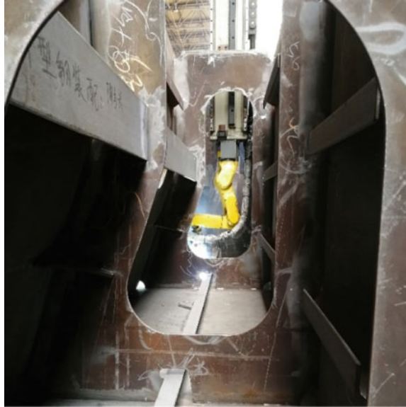
(a) Robot vertical welding
