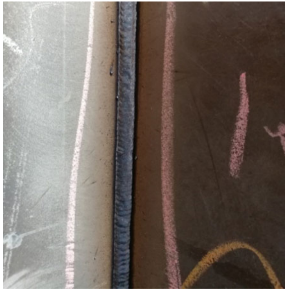
(b) Forming of vertical welding joint
