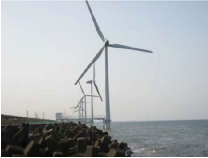
Fig. 9 Photograph of the Kamisu (Hasaki) wind farm following the 2012 Tohoku earthquake
