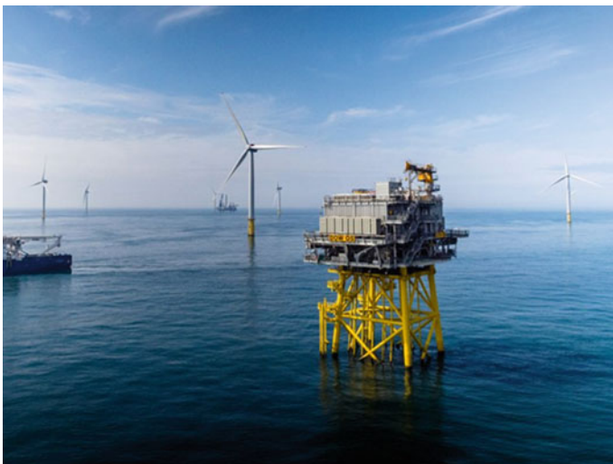
Fig. 3 Aerial view of Dudgeon wind farm. Photo Jan Arne Wold, Equinor
