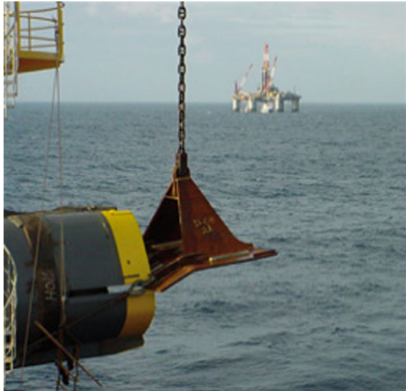
Fig. 18 SEPLA being inserted into suction caisson slot
