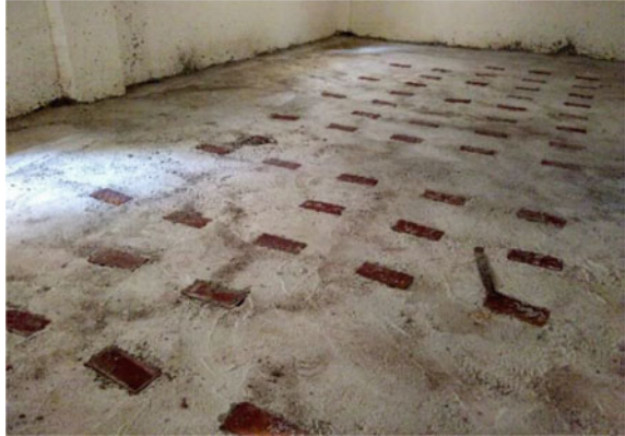
Fig. 2 Strong concrete floor in the foundation laboratory
