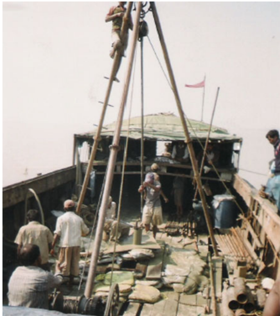
Fig. 2 Subsurface exploration in progress
