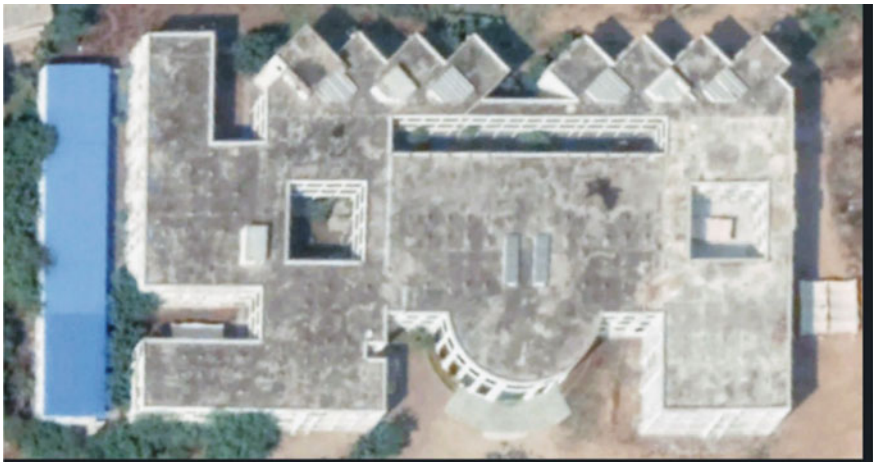
Fig. 2 Rooftop area of the campus considered taken from “Google Earth” (2019)
