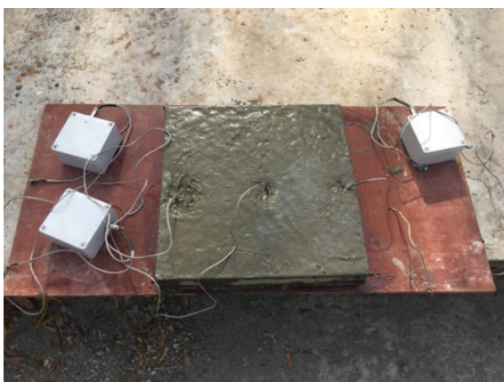
Fig. 4 Placement of sensors in a square manhole cover
