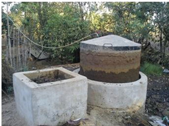
Fig. 1 Biogas plant setup
