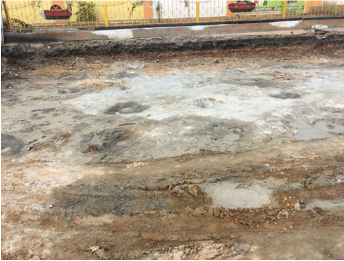
Fig. 1 Stabilization of expansive soil in Salem new bus stand
