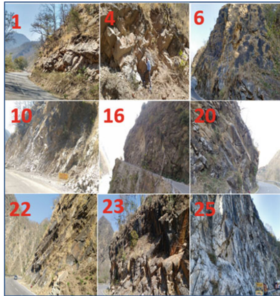
Fig. 2 Field photographs of some studied slopes
