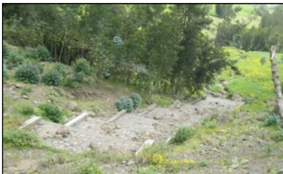
Fig. 18 D/s side valley slope protection works done at pipe culverts in Ethiopia
