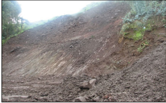
Fig. 15 Hill slope done at project roads in Ethiopia
