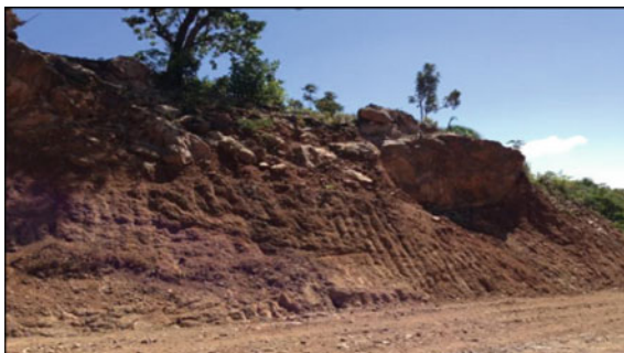
Fig. 10 Hill slope excavation along “Adiremet–Dejena–Dansha”
