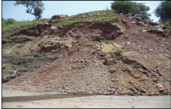
Fig. 5 Landslide from hill slope along “Adiremet–Dejena–Dansha”
