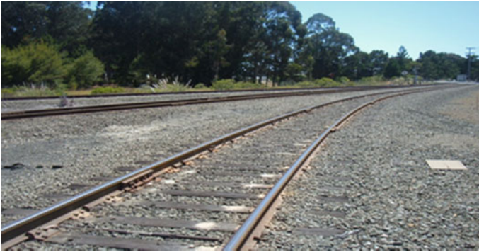
Fig. 1 Lateral spreading of ballast in ballasted railway track (sourced from Hussaini et al. 2013)
