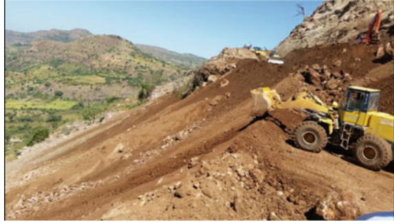
Fig. 11 Construction of hill road along “Adiremet–Dejena–Dansha”
