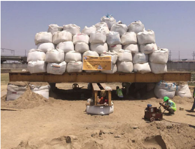
Fig. 4 Single-column load test set-up
