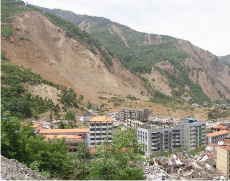
Fig. 2.1 The Wangjiayan landslide triggered by the 2008 Wenchuan earthquake
