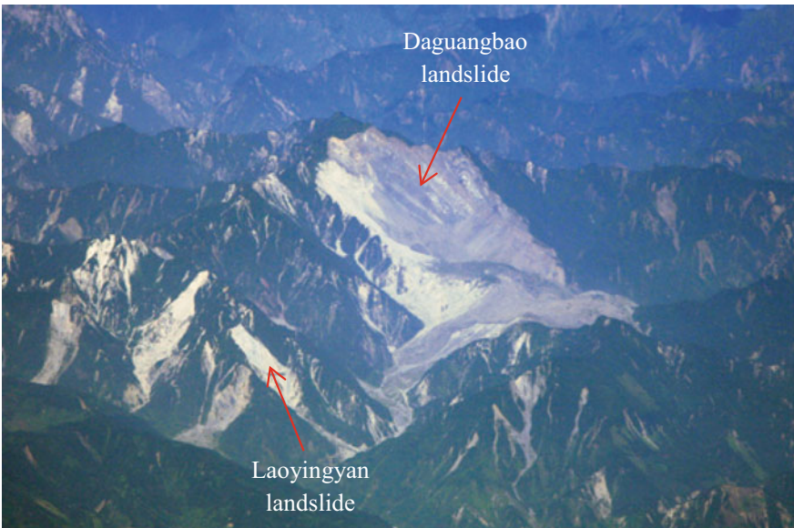
Fig. 2.2 The Daguangbao and Laoyingyan landslides. Photo taken by Huang and Fan [10]
