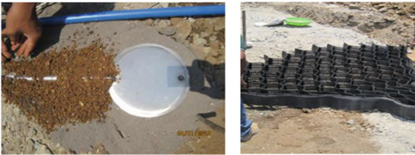
b Instrumentation and construction of reinforced section
