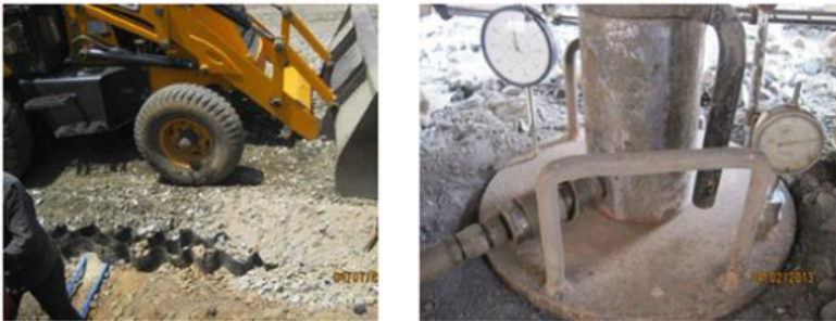
c Construction of geocell reinforced GSB layer and load test
