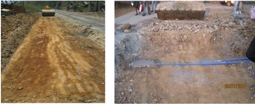
a Excavation of existing pavement, preparation of site with instrumentation (TPCs)
