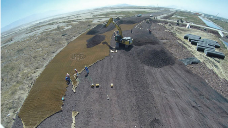
Fig. 15.1 Soil stabilization of poor subgrade with Neoloy Geocells. Photo credit Innovater
